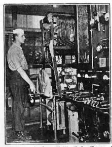
Control Panel of 20 K.W. Tube Transmitter at NAA, the U. S. Navy Station at Arlington, Va.
