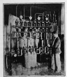
Rectiper 1 uve Unit of 80 K.W. Tube Transmitter at San Diego.
