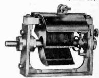
and are guaranteed to be accurate within 1 per cent of their rated capacitances. They are small and compact and built to a tolerance of .001 in. With their one-hole mounting they can be placed either horizontally or vertically. The rotor is grounded.
