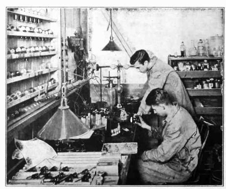
Developing a New Long-Life Filament for a Low-Temperature Power Tube.
