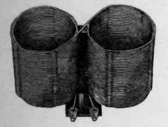
minimum of supporting insulation in its field decreases power losses. It can be mounted in any position as its external field is so slight that close spacing is possible without appreciable interaction. It will work satisfactorily with any high grade .00035 mfd, variable condenser.
