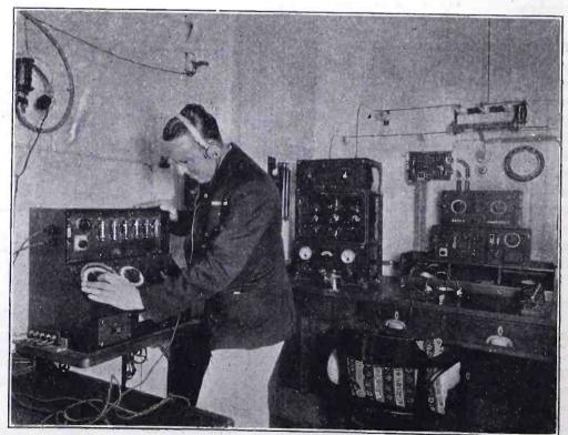
11/2 K. W. Tube Transmitter on S. S. "Majestic" showing Operator Brunt using "D. F." Radio Compass
