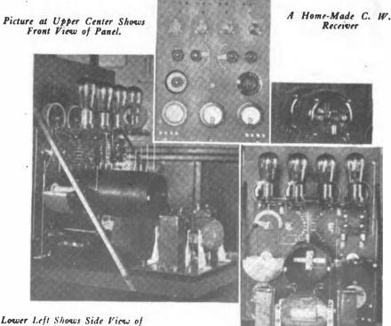
Lower Left Shows Side View of Panel Rear. Lower Right Shows Full-on View of Panel Rear.
