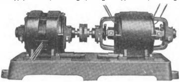
Fig. 71. Double Commutator Generator
