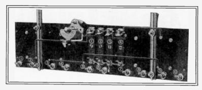
Bottom view of sub-panel illustrating correct wiring.
