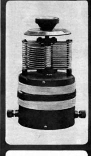
Another form of the wave trap spoken of in this article. Here the variable condenser is mounted high above the eoil so as to be kept away from the magnetic fields
