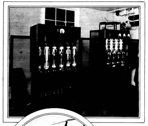
Photo at top is the inside of KDEF. the ground station of the night air mail service at Omaha, Neb. the left is the unit which rectifies 6600 volts, alternating current into 2000 volts direct current, for the speech amplifiers and modulators at the right
