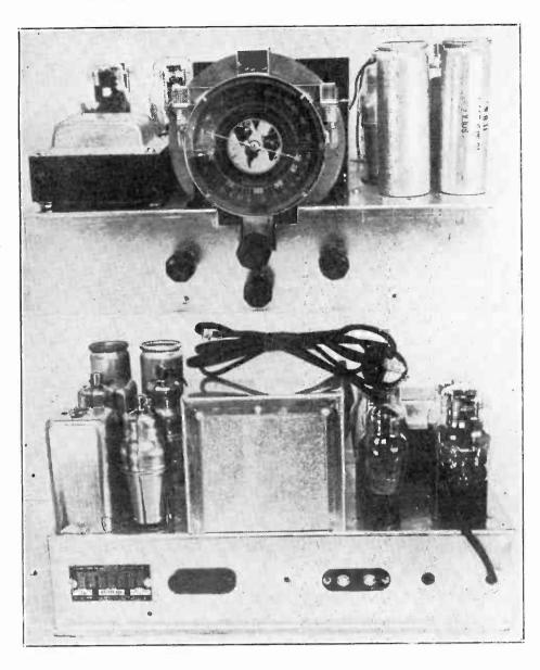
Close quarters for controls sometimes are unavoidable, especially where there is limited space at the console opening. Therefore with a band switch, volume control and tuning knob, if a tone control is to be added it may be put under the tuning knob, as in this Air-King receiver. Acc cable projecting from rear should be protected by grommet or eyelet.
