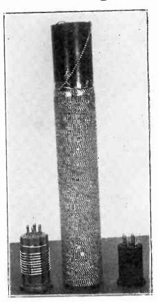
At center is not the Solenoid Sphynx of Egypt, bodyguarded by Hammarlund coil and form, but simply a 2-inch diameter wound with all the No. 18 (bell) wire directed to be put on for constituting the inductance for a power line r.f. filter. Expert who recommended the number of turns reports slide rule slipped.
