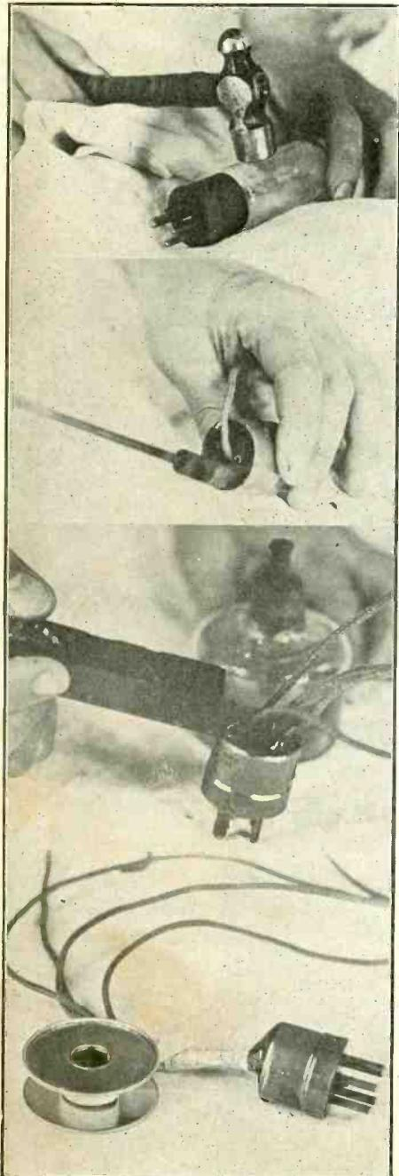
FIG. 1, the breaking of the glass envelope. This is followed by the soldering of lamp cord to the base tips of the tube. (Fig. 2). Sealing wax fills up the shell. (Fig. 3). Next (Fig. 4) the four wires are braided.
