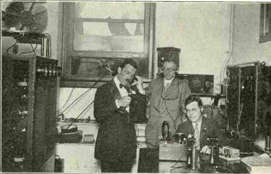
FIG. 5, what the inside works of WNYC, the New York City Municipal Broadcasting Station, looks like. To the extreme upper left is the antenna inductance. The man seated is operating a wavemeter. To his left is a key and a buzzer.
