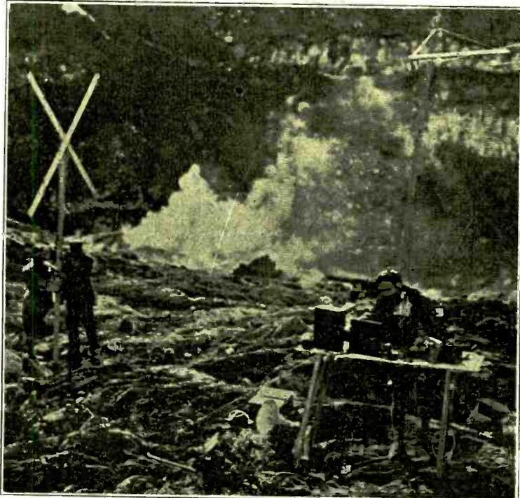
THE ACTUAL TEST of radio reception within the crater of Mt. Vesuvius, with smoldering recesses at hand and death-dealing gases filling the air, proved that reception on a loop was impossible within the eruptive zone. The loop was strung around the white cross shown in the photo. Note that the two men supporting the loop wear a gas mask, as does the man attempting to tune in a station. (International Newsreel)
