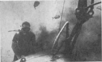
At 110 foot level, diver Ed Davies inspects cables connecting Sea Spider's underwater sphere to telemetering buoy at surface. The many inquisitive fish bring other, unwelcome visitors, dangerous sharks and toothy barracuda, to the experimental "inner space" anchorage.
