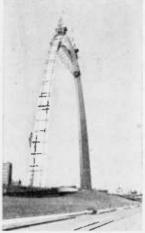
Highest U. S. monument, the 630-feet, \$30-million Gateway Arch rises majestically above St. Louis skyline, its welded joints 100 per cent inspected with the aid of nuclear energy emitted by a radioactive isotope. Its welded panels are designed to withstand winds of more than 150 miles an hour.
