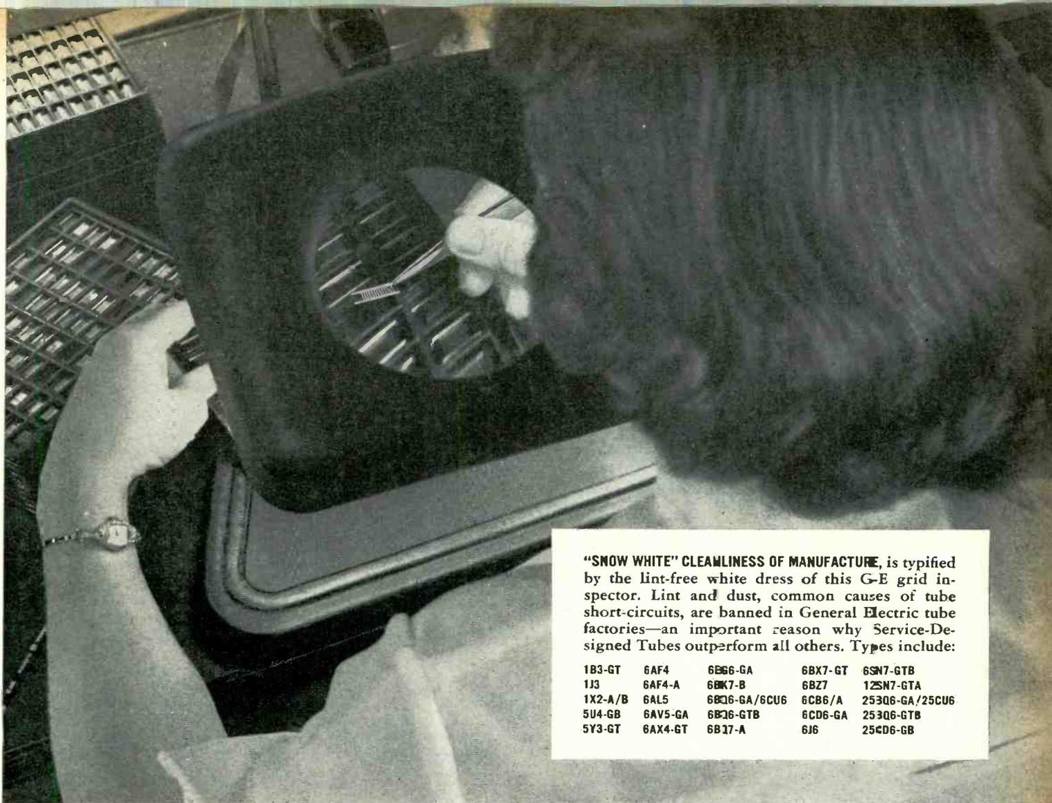
"SNOW WHITE" CLEANLINESS OF MANUFACTURE, is typified by the lint-free white dress of this G-E grid inspector. Lint and dust, common causes of tube short-circuits, are banned in General Electric tube factories—an important reason why Service-Designed Tubes outperform all others. Types include:
