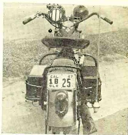
Rear view of complete assembly showing control head, mike, xmtr-receiver, and antenna.
