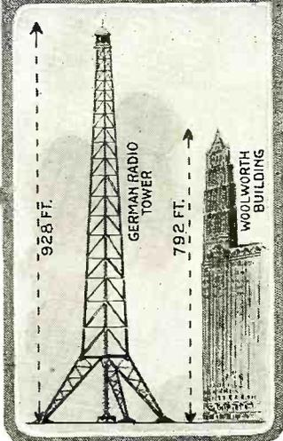
The steel aerial tower at Konigsrueterhausen, near Berlin, Germany, just erected, is 928 feet high; with its mast it will reach higher than the Eiffel Tower. A one-passenger elevator runs to the top.
