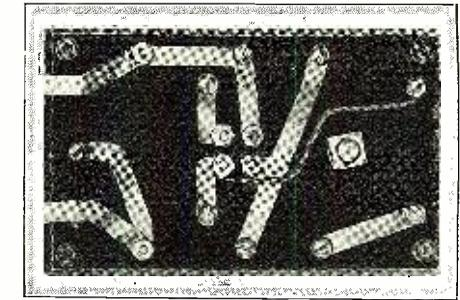
Several years ago strip connections were tried instead of wire in order to introduce capacity at certain points. The bottom view of a one-tube set built in 1920.
