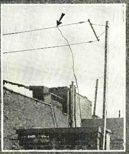
Above: The lead-in should have been taken off from the end of the aerial and the aerial itself guyed with ropes. Right: This ribbon aerial is well fastened to the pipe with a piece of rope but is not insulated.
