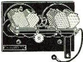
Radio Devices, Woonsocket, R. I. This unit has a method of connecting condensers so that "single-control effect" is obtained.
