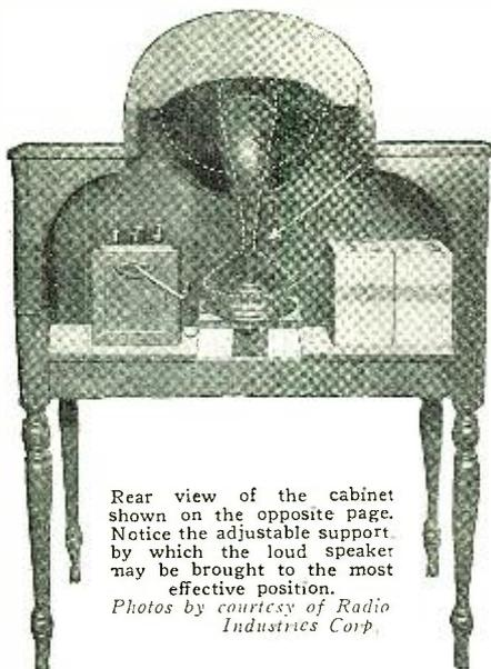
Rear view of the cabinet shown on the opposite page. Notice the adjustable support by which the loud speaker may be brought to the most effective position.
