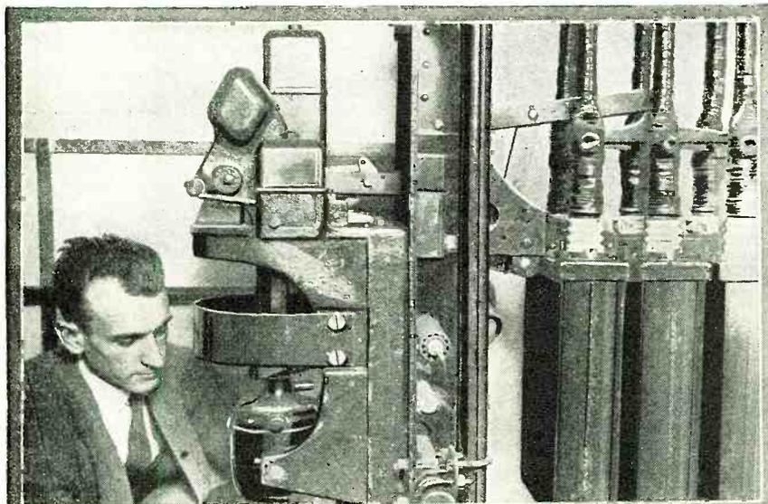
**WATER COOLER FOR VACUUM TUBES.** This huge water cooler, which is capable of cooling 100 gallons of water per minute, is used for the purpose of keeping the giant vacuum tubes used in the transmitter at an operating temperature. This is necessary because the great power which is needed to operate these tubes would ruin the comparatively delicate elements in a short time.
