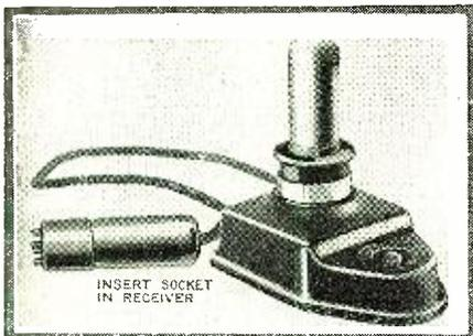
This compact instrument gives a quick, qualitative test of tube functions which would require half a dozen accurate meters to duplicate quantitatively.
