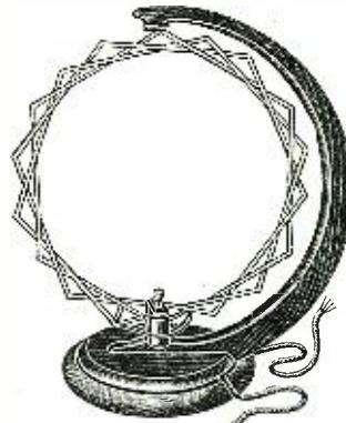
ORATORIES for test, by Eclipse Radio Laboratories, Rock Island, Ill. It is of special construction, being wound in the most approved low-loss, basket-weave form, thus giving a high degree of efficiency and enhanced directional property.
