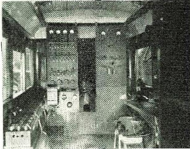
Fig. 2. At the right may be seen in interior view of the portable broadcast station, the exterior of which is shown at the bottom of the page. At the left are the battery racks. The two long panels control the generators and the transmitting tubes.
