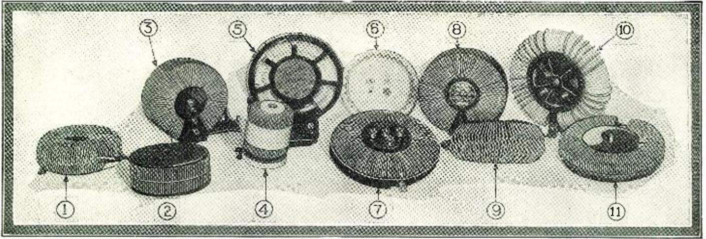
Different commercial makes of toroids: 1, Orbit; 2, Nolte Circoils; 3, Bremer-Tully; 4, Radio Foundation Torocoil; 5, Thorola; 6, Summit; 7, Erla Circooids; 8, All-American; 9, Peri Coil; 10, Naxon; 11, Wybo Hexoids.
