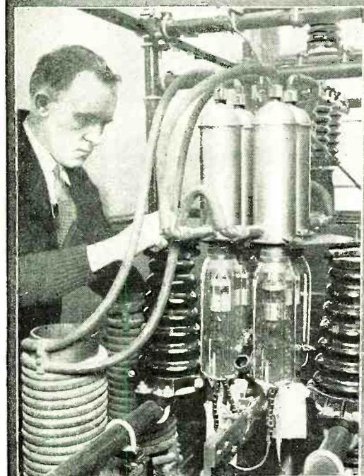
**A MOTOR - OPERATED OIL SWITCH.** Above is shown one of the large switches, which is located in a house of its own and controlled from the central switch board. This switch is operated by a remote-control switch, which closes a circuit starting the motor shown at the bottom of the photograph. By running the motor in the opposite direction the switch is opened.
