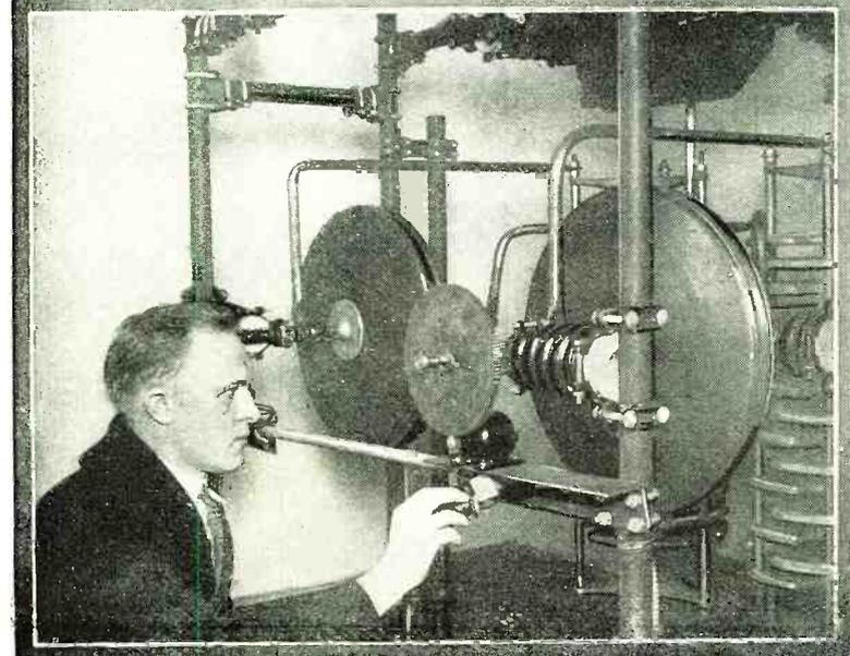
**GIGANTIC VERNIER CONDENSERS.** On the left is shown a pair of air condensers which are used for sharpening the tuning of WJZ. They operate by varying the separation between the plates and are verniers to the big condensers, the plates of which can be seen in the extreme right background. The verniers are operated electrically by small electric motors. Photos © Kadel & Herbert.
