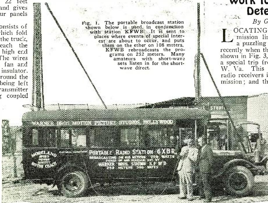
Fig. 1. The portable broadcast station shown below is used in conjunction with station KFWB. It is sent to places where events of special interest are about to occur, and puts them on the ether on 108 meters. KFWB rebroadcasts the programs on 252 meters. Many amateurs with short-wave sets listen in for the short-wave direct.
