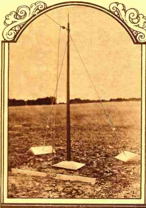
**ONE OF THE GROUND PLATES OF STATION 5XX.** The newest of England's broadcast stations has a unique ground. Surrounding the station are plates, buried as shown in the photograph above. The wire connecting them to the transmitter is carried from the plate to the insulator on top of the 15-foot pole.
