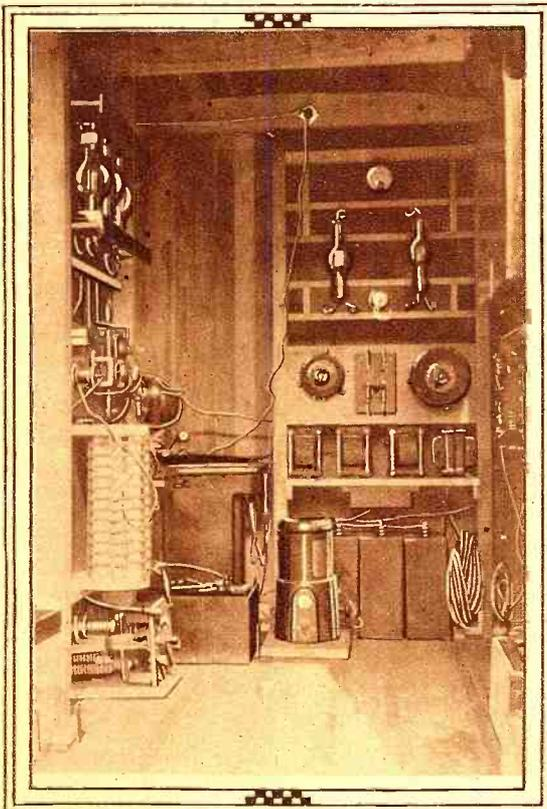
**REAR VIEW OF THE KDKA RELAY TRUCK.** The supports for the antenna are behind the left door and the antenna is slung under the floor of the truck.
