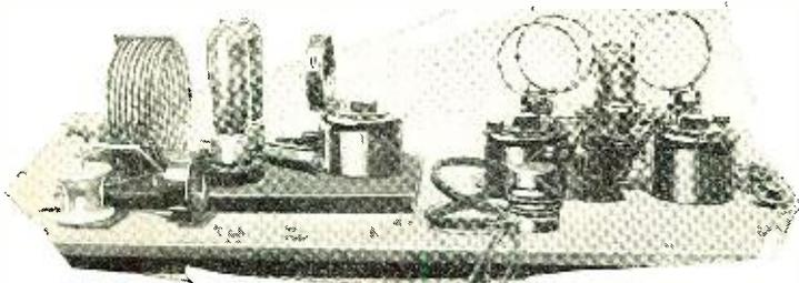
The radio apparatus which made the Amazon neighbor to the Bronx. Note the extreme simplicity and lightness of the outfit.
