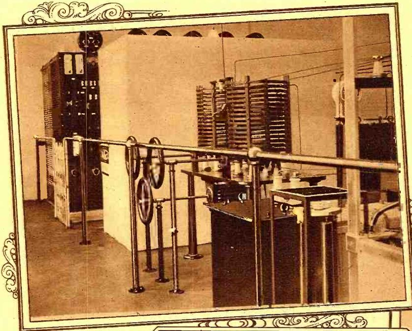
← **TRANSMITTING ROOM.** Here are shown the high frequency inductance, the condenser case and the output transformer. The station has a rated power of 25 KW.
