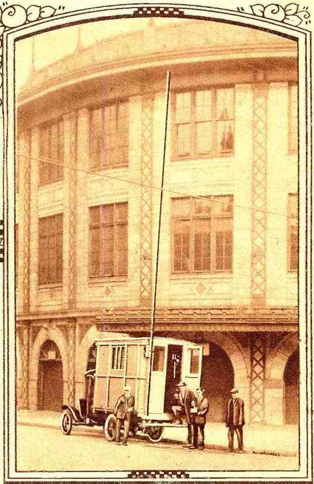
**A COLLAPSIBLE ANTENNA.** The antenna of the portable relay station used by KDKA as a pick-up station. The antenna is a collapsible jointed copper rod of the vertical oscillator type and is shown in the above photograph attached to the truck that houses the station.
