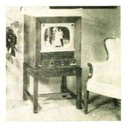
The first of this firm's line to use the 16-inch picture tube, this television consolette ensemble (receiver and matching table) has the convenience and flexibility of a separate instrument and table. Has dual dynapower loudspeakers, 12 TV channels with separate circuit for each, Gruen circuit for picture synchronization, and automatic gain control.
