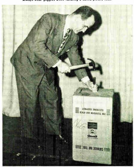
To discard — seal cathode-ray tube in a carton, then drive a crowbar or blunt instrument through carton top.
