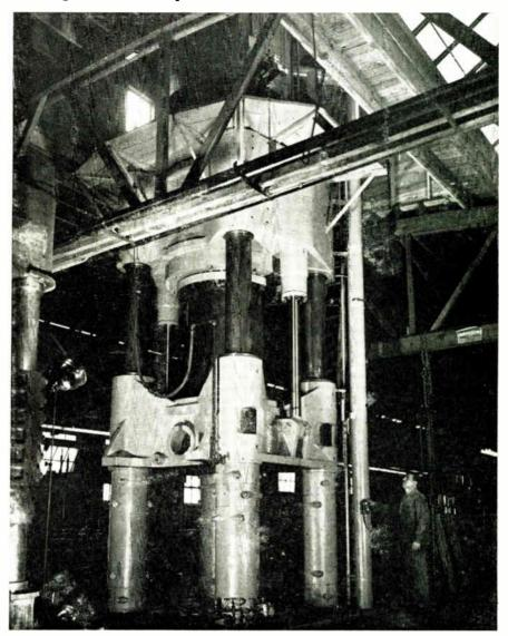
This operator clicks a switch, the 2,000-ton hydraulic press goes to work, and in six minutes another plastic cabinet is ready for the television production lines of the Admiral Corp.
