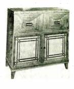
A new modern blonde console radio-phono, model 148CO. The chassis, with the Crosley "floating jewel" tone system, has 18 watt power output, 12" permanent magnet speaker with 12 tubes, one rectifier and 1 tuning indicator.
