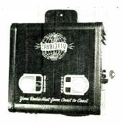
Called Tradio-ette, this 6-tube receiver is said to be the smallest coin-operated radio in the world, measuring only 7½" wide x 71/2" in length and 5" deep. After being laboratory and location tested for almost a year, this unit is now in full production. Other features are: a three-gang condenser, present maximum volume which restricts program to individual booth, simple plug-in installation, timer, pick-proof lock and the "Tradio-tenna, which eliminates the need for outside aerial.
