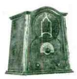
Stewart-Warner Corp. introduces the Metropolitan Midget, a walnut cabinet Job 14% ins. high and 1214 ins. wide, complete with tubes, at \$34.95, Specially designed for use in metropolitan areas, for reception within 200-mile radiin. Equipped with new S-W 7-tube rhassis and specially designed dynamic speaker. Employs both variable mit and pentade tubes.
