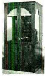
An automatic coin-controlled voice recording machine, invented by J. E. Byrnes, and manufactured by the Speak-A-Dise Corp., is presented especially for use in hotel lobbins, railroad depots, steamships and unmsement parks. It dispenses a 6-inch Remsen disc in a mailing carton, the apparatus coming with or without booth. A playback machine allows customers to hear their records.
