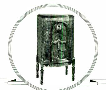
MODEL 17—Lowboy walnut console of distinctive design. Superheterodyne, 9 tubes. Color tone control, Brunswick Uni-Selector, automatic volume control, dynatron oscillator, turret type tuning condenser, 12" super-dynamic speaker, two pentode tubes in output stage and power detector. Dimensions 414" high, 214" wide, and 134" deep. List price, complete with Brunswick tubes . . . \$149.50
