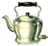
An electric hot water kettle, bearing the "Universal" trademark, is presented by Landers, Frary & Clark. Of aluminum construction, equipped with ebonized handle and knob and 6 feet of heater cord, this appliance has a 3-quart capacity and a 1,000 wattage. Its packed weight is 4 lbs., and it is packed one in a carton, or three in a unit package. The catalog number is E9263.
