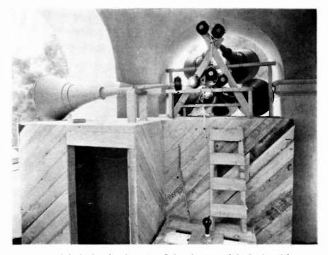
A rear view of the loudspeaker clusters installed in the tower of the Foods and Beverage Building. The low-frequency speakers are installed underneath the horns in the enclosed structures. The insides of these structures are acoustically treated to prevent resonance.
