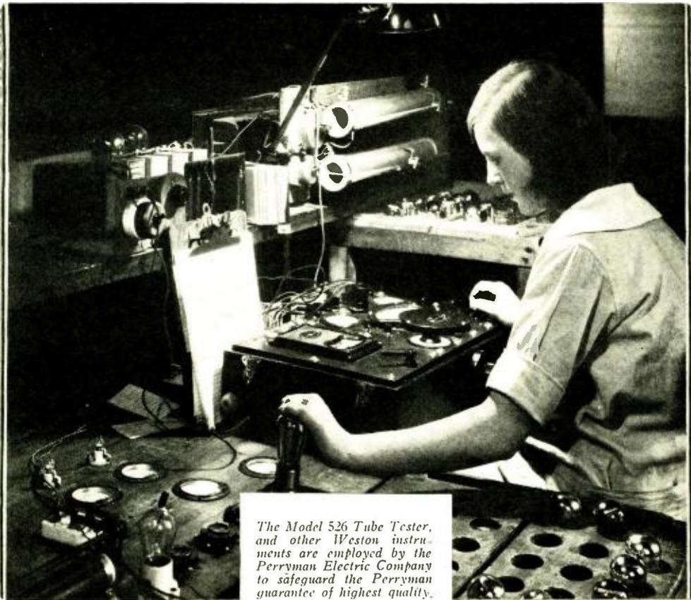
*The Model 526 Tube Tester, and other Weston instruments are employed by the Perryman Electric Company to safeguard the Perryman guarantee of highest quality.*
