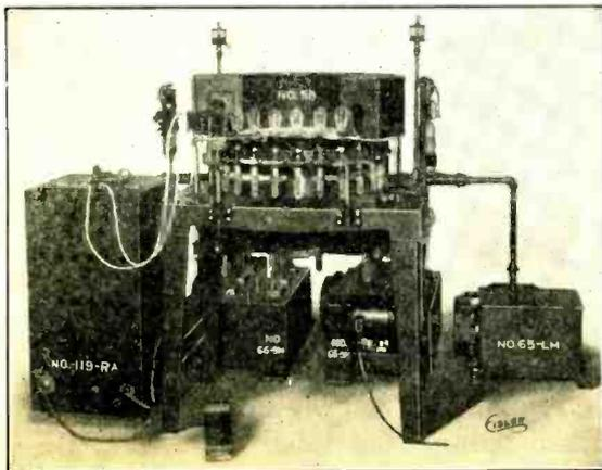
A complete Eisler 24 head A.C. automatic exhaust machine installation. A battery of high vacuum pumps is connected directly to the machine.
