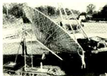
SATELLITE RECEIVING ANTENNA being mounted on posts in authors' backyard. To find out what's being broadcast and the frequencies, turn to page 47.
