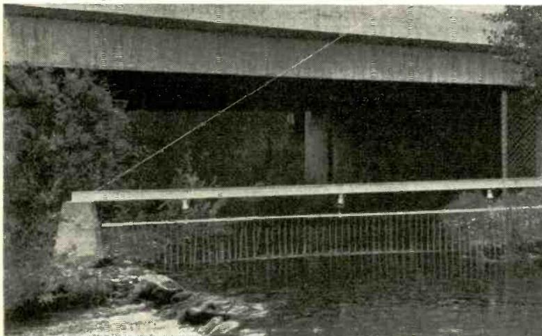
Fig. 2—Electrode system of an electronic fish screen at the intake for an irrigation district.
