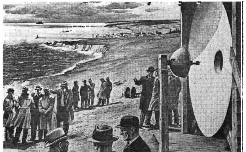
An artist's conception of the world's first demonstration of communication by microwaves in 1931. This commercial link between Dover England, and Calais, France, was designed by European subsidiaries of International Telephone and Telegraph Corp.
