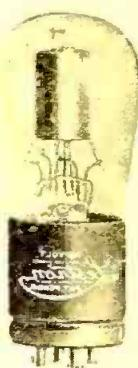
Their new tube operates equally well on any 110 volt supply having either direct or alternating characteristic. It contains two electron emitting surfaces, which result in a far richer electronic emission per unit of surface than is obtained in the present storage battery type tube, which in turn tends to prevent the possibility of overloading.
