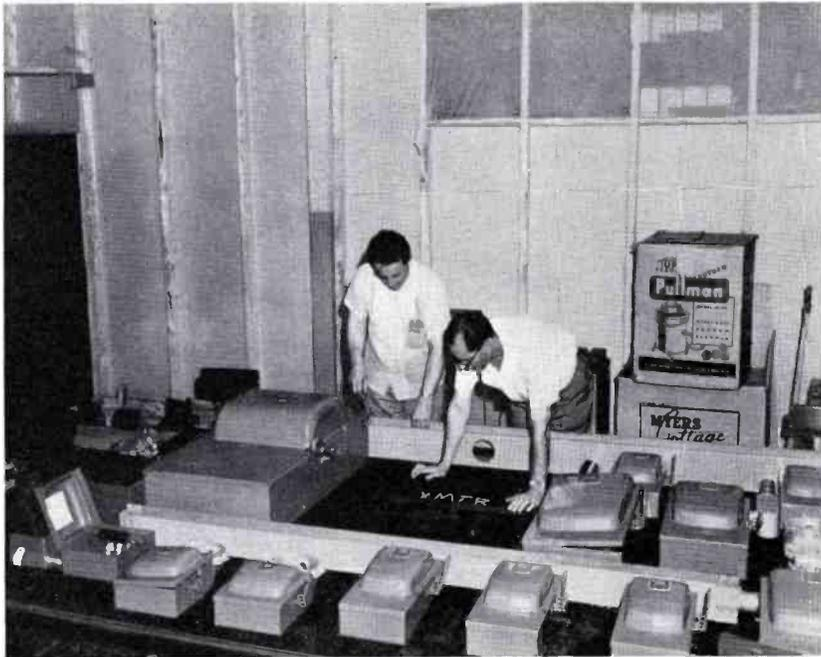
FIG. 12. Power load center is carefully laid out and preassembled. Other units usually assembled on the job, such as water systems and air ducts, were also prefabricated.
