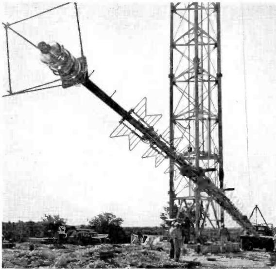
RCA TF-12AH 12-section Superturnstile starts its long journey to the top tower platform. Upper left corner shows detail of beacon and lightning protector.
