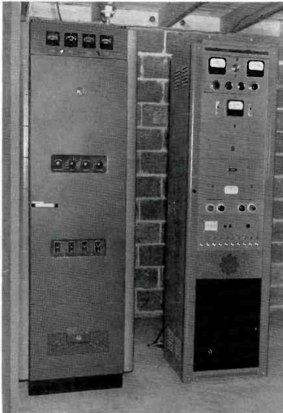
RCA BTA-250M, 250 watt transmitter (left) with RCA BTR-5A remote-control rack (right) constitute the unattended remote-control equipment.
