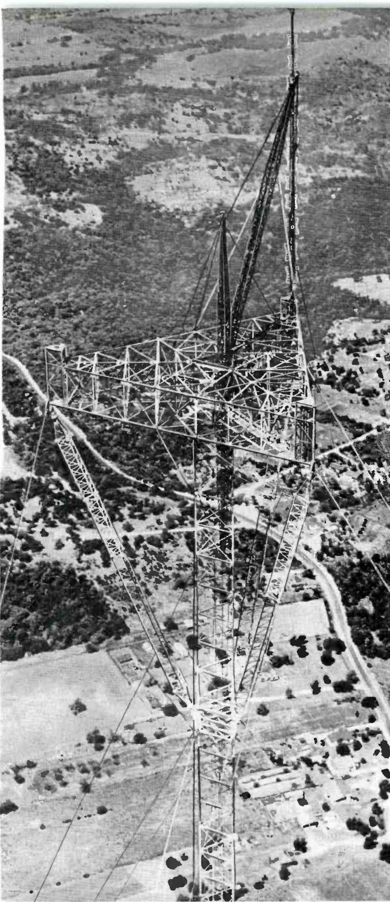
ABOVE—Nearing final construction, this aerial view, taken by the Dallas Morning News, shows RCA 12-Section Superturnstile Antenna of WFAA-TV being mounted.
