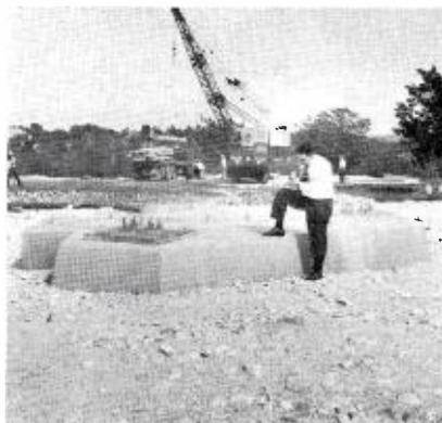
One of many typical guy anchor piers with steel plates in place.
