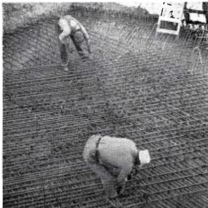
Placing reinforcing steel in tower foundation pits. A total of 35,000 pounds of steel was used for this purpose.
