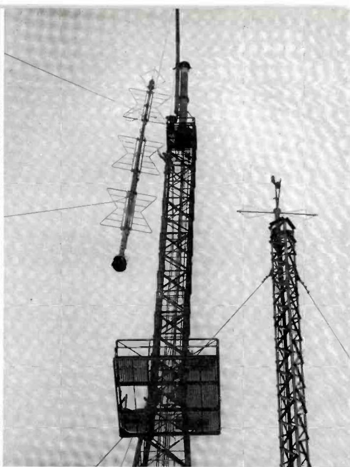
FIG. 4. The RCA TT-3B Superturnstile Antenna nearing the top of the tower. The temporary antenna can be seen at the right, foreground.
