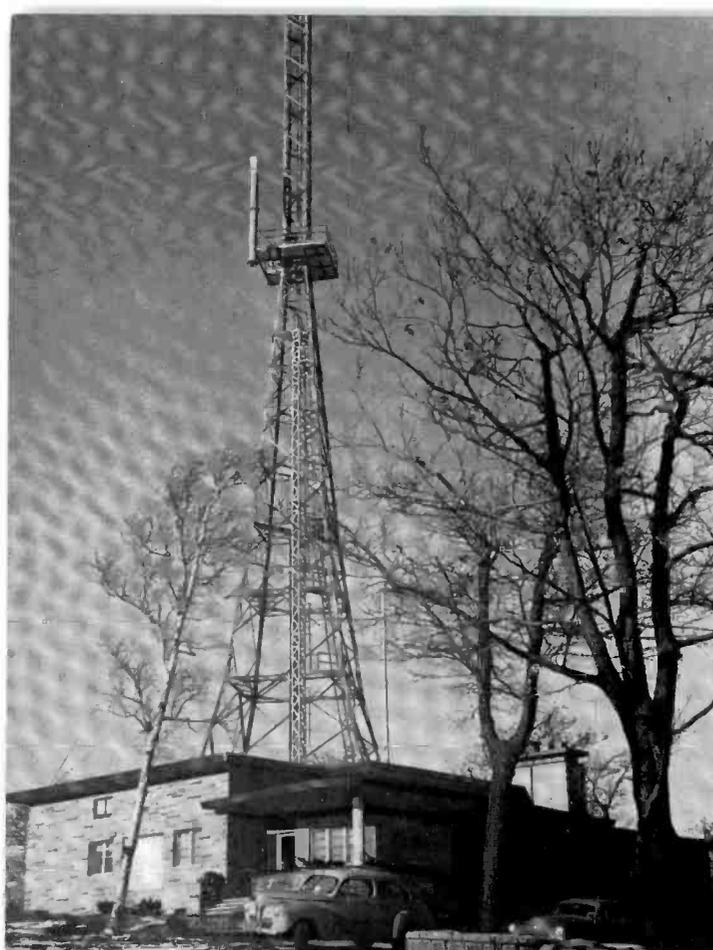
FIG. 3. Two-section heavy duty Pylon passing microwave platform. Constant cross-section of tower from this point to the top is for channel 6 Supergain Antenna.
