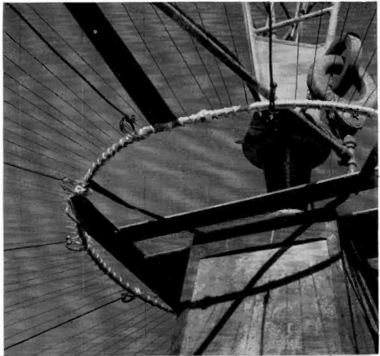
FIG. 7 (opposite page). Overall view of the elevated ground screen installed around each of the KTBS towers. This arrangement provides a stable antenna impedance because changes in vegetation or ground water in the critical area around the base are minimized.
