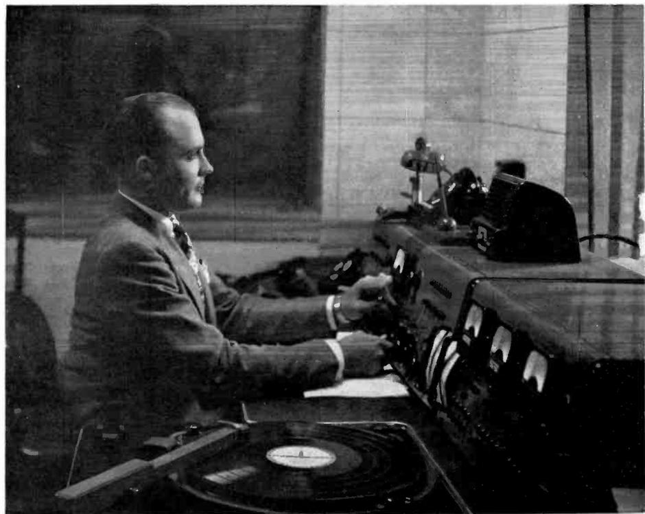
FIG. 4 (right). Marvin L. Perry, Chief Studio Control Operator, at the console in the AM control booth. Equipment—all RCA—includes a 76-C Console, a BCS-1A Master Switching Console, 70-D Turntable and LC-1A Speakers. The FM control room, directly above, is similarly equipped.
