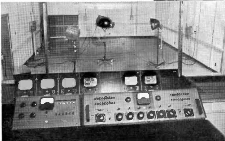
**KGO-TV.** Video control-room equipment at KGO-TV—as in all the other ABC-TV stations—is completely RCA. KGO-TV also uses RCA field cameras, microwave relay equipment, field truck, sync generator, studio cameras, film projectors, slide projectors, film cameras, turntables, microphones and an RCA Superturnstile antenna.
