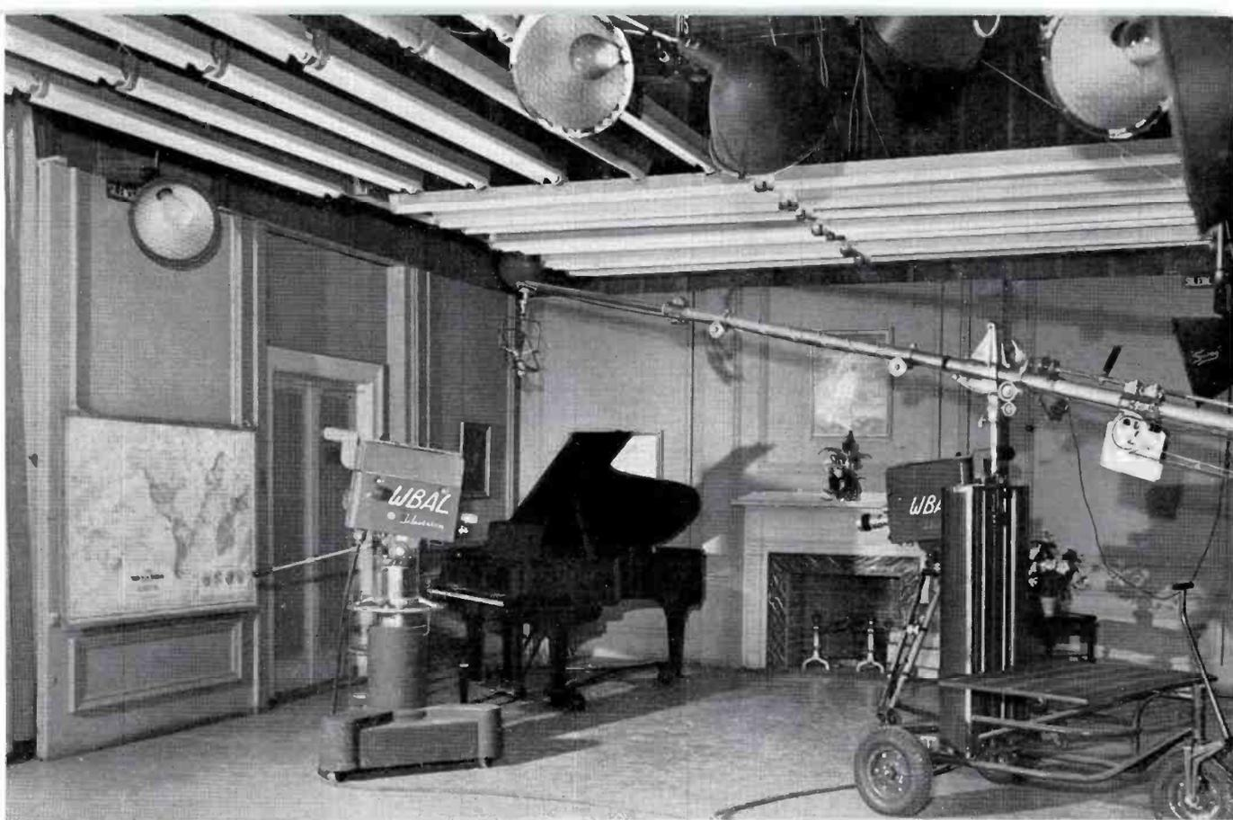
FIG. 6. Newly installed banks of fluorescent lights, used in conjunction with incandescent flood lamps, provide the illumination for Studio H. Photo shows one corner of the well appointed "Georgian Room."
