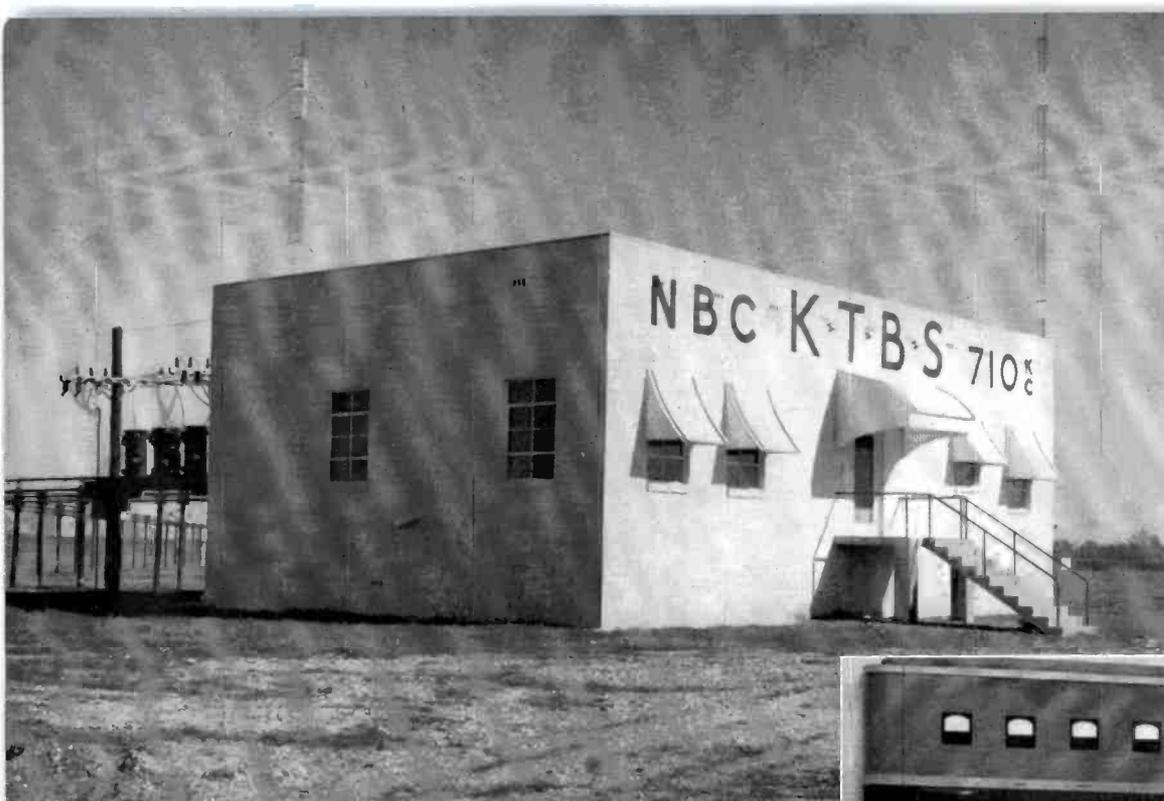
FIG. 1 (above). KTBS' new transmitter building is located 14 miles northwest of Shreveport. Floor of the fireproof building is five feet above ground level so that equipment is safely above possible flood waters.
