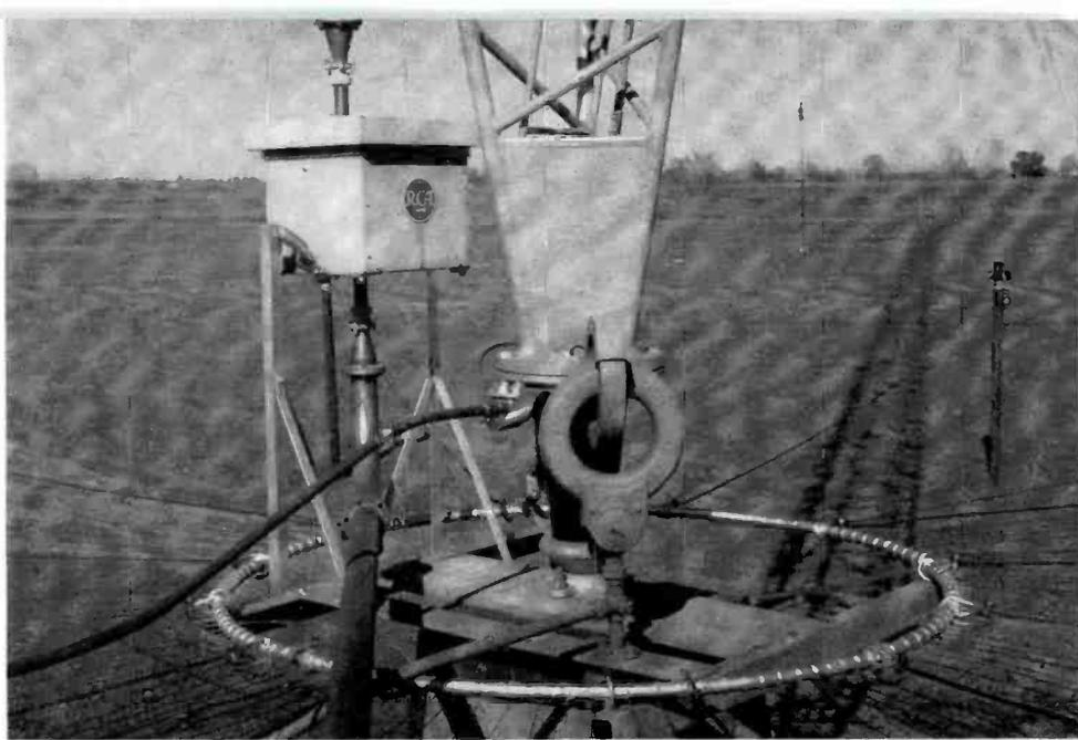
FIG. 8 (right). This close-up view of the base of one tower shows the BAF-4A FM Isolation Unit (in square box) and the Austin Transformer (large open coils) used to isolate the tower lighting circuits.
