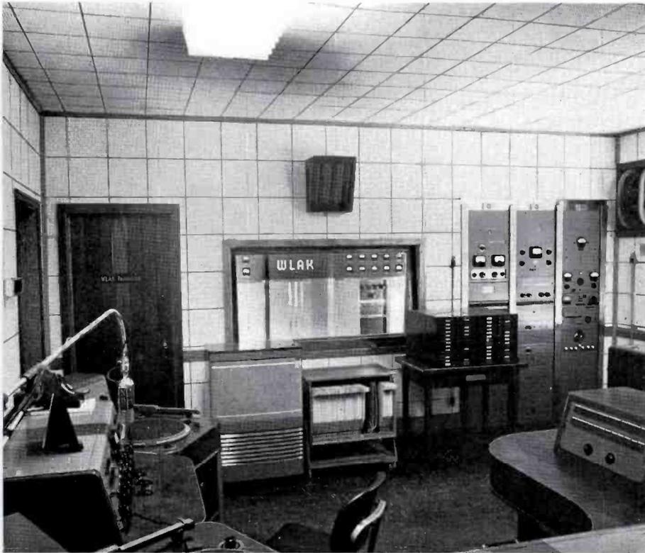
FIG. 1 (above). The WLAK, 1 KW transmitter is visible from window of central control room. Note that monitoring test and audio racks, as well as studio control consoles are all easily reached.
