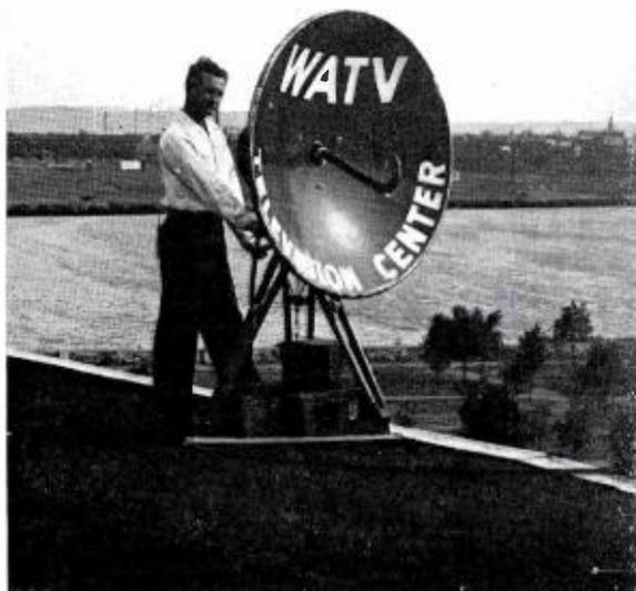
WATV, like nearly all stations telecasting baseball, uses RCA Microwave equipment to relay video signal to studio or transmitter. In many cases roof of grandstand provides necessary height for transmitting parabola.
