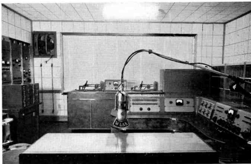
FIG. 3 (above). View from WLAK studio, looking into control room. Visible at rear is the WLAK dual-recorder which employs type 73-B professional unit.
