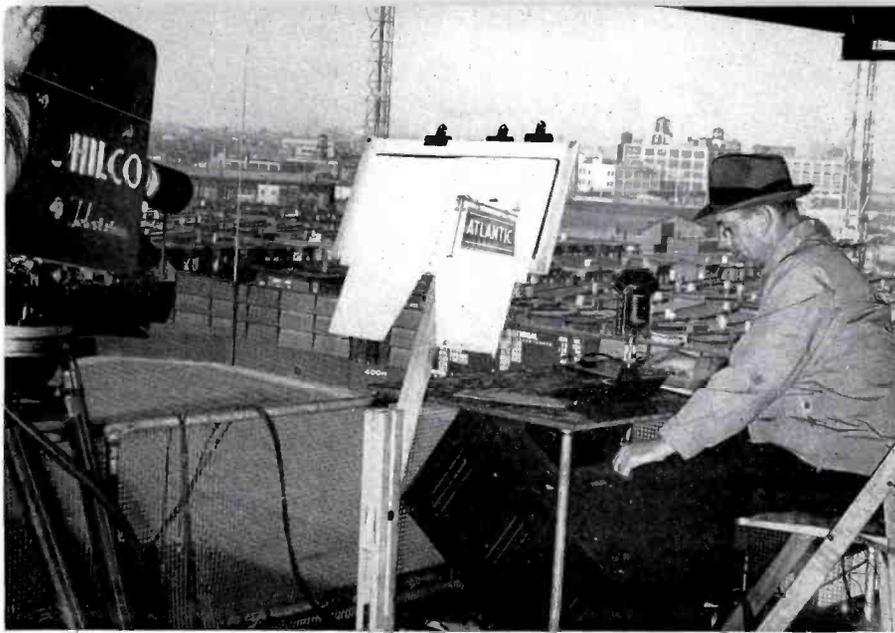
FIG. 22 (left, above). One arrangement for originating commercials at the park is illustrated by this WPTZ setup at Shibe Park, Philadelphia. Charts, arranged for easy turning, are mounted on an easel near the No. 2 Camera, which can be focused on this as announcer sitting at table reads continuity. Note monitor mounted on table does not obstruct announcer's view of field.
