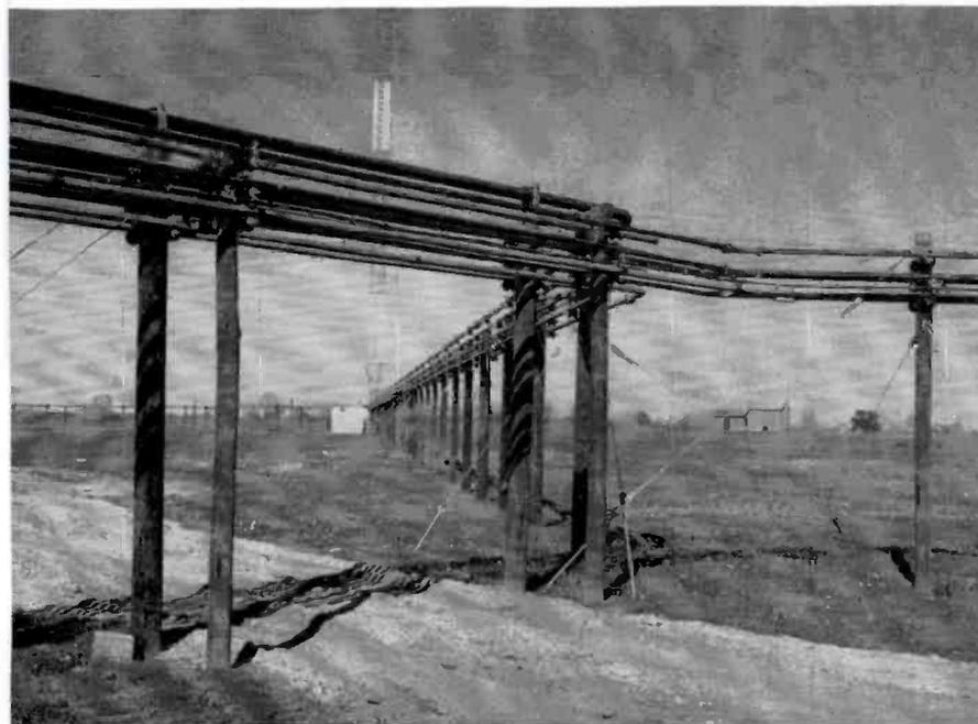
FIG. 6. This is another view of the transmission line branching point. Because separate feed systems are used for day and night transmission there are two concentric lines to each tower. The large line at the top is the concentric line feeding the FM antenna at the top of No. 3 tower.
