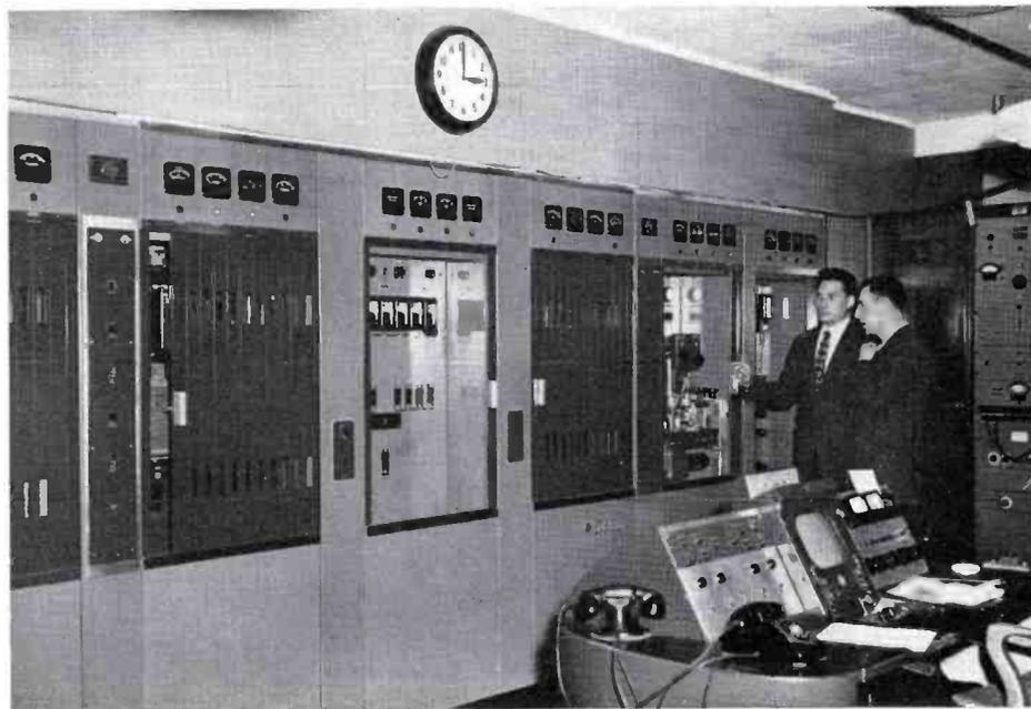
FIG. 8. The 12-kilowatt transmitter installation. The false wall has been removed to provide space for the extra cabinets.
