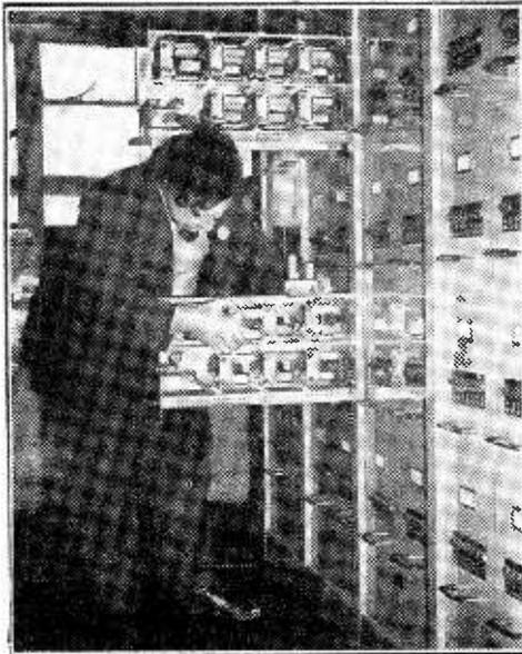
A technician replaces an output unit into the radio distribution unit of a channel used by controllers speaking to aircraft. (See "Air Traffic Control".)
