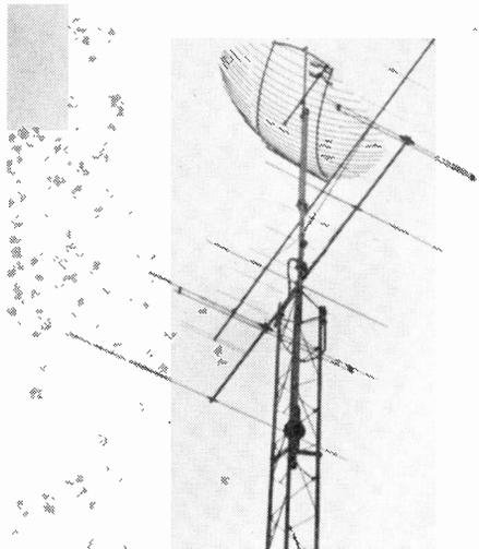
The top section of Roger's present aerial structure, with the u.h.f. paraboloid atop.
