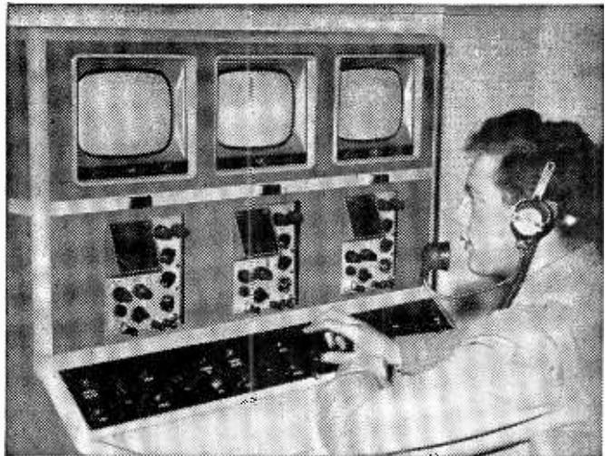
The Remote Control Console for Marconi Broadcast Vidicon cameras which is now installed in Havelock House, Belfast. It was designed and built by Ulster Television engineers.
