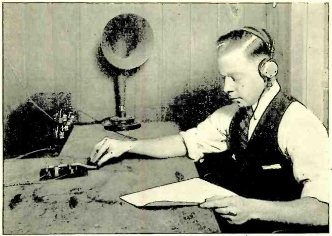
From a photograph made for POPULAR RADIO HOW TO LEARN THE CODE The man in the picture is sending himself code letters on a buzzer which he hears in the headphones. This is one good way to practice the receiving speed required for an operator's license.
