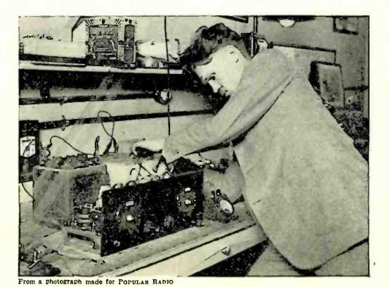
HOW TO OBTAIN GREATER ECONOMY IN SUPERHETERODYNE OPERATION FIGURE 5: It is possible to effect a great saving in "B" battery consumption by reducing the plate voltages of superheterodyne receivers. In many cases such a reduction can be accomplished without in any way reducing the efficiency of the receiver.
