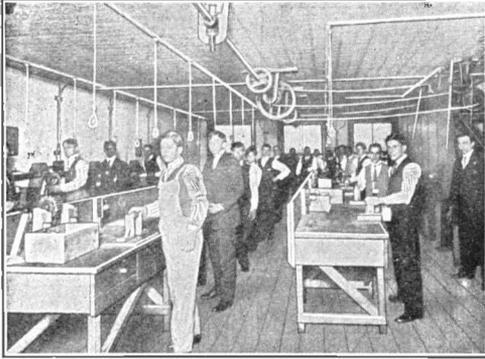
STUDENTS PERFORMING PRACTICAL WORK IN ARMATURE WINDING AND PATTERN MAKING
