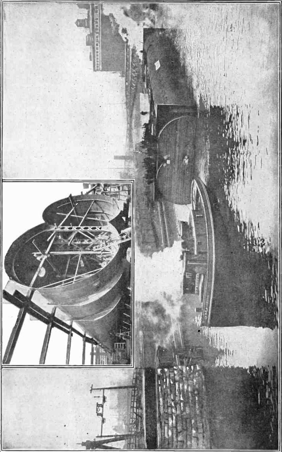
GIANT TUBES FOR ELECTRIC RAILWAY TUNNELS UNDER THE CHICAGO RIVER, AND HOW THEY WERE FLOATED INTO POSITION
