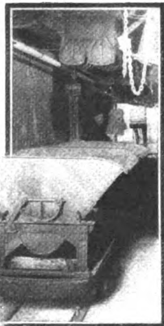
Front of One of the Boilers Showing How the Coal Is Led Down Until Within the Clutches of the Automatic Stoker
