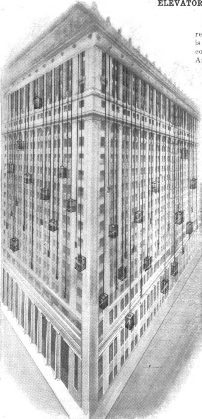
Twenty-three Elevators in a Single Building. Each Like a Bucket Hung in a Well
