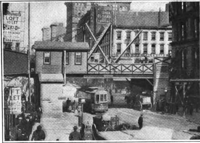
The Shaft in Broadway and Canal Street, Looking North on Broadway
