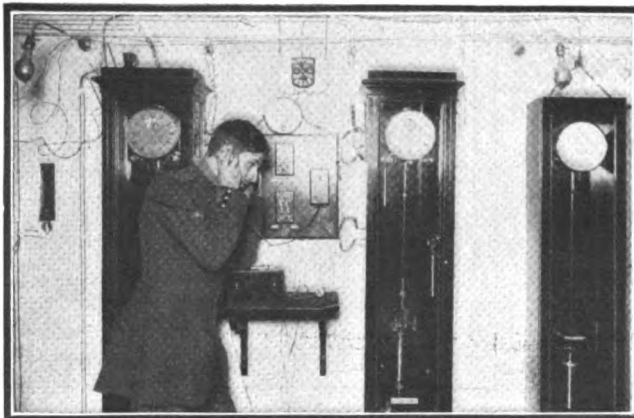
Operator Brill at the Automatic Apparatus Which Opens and Closes the Signal Circuit
