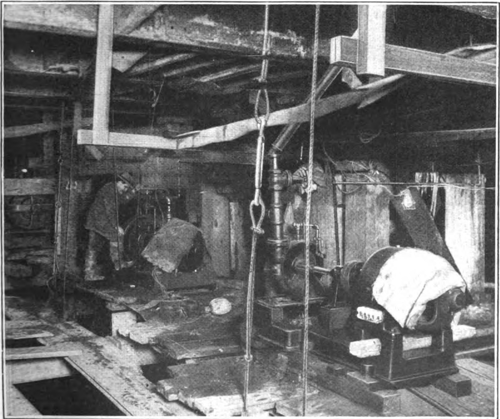
Three of the Motors and Pumps that Are Lifting 20,000,000 Gallons of Water a Day Out of the Old Canal
