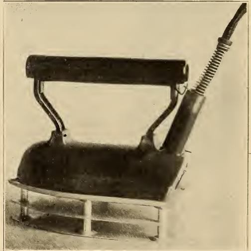
FIG. 32. THE ELECTRIC FLATIRON — AN EXAMPLE OF THE HEATING EFFECT OF ELECTRICITY.
