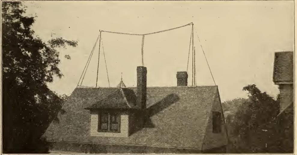
FIG. 22. DOUBLE-ENDED "T" TYPE ANTENNA.
