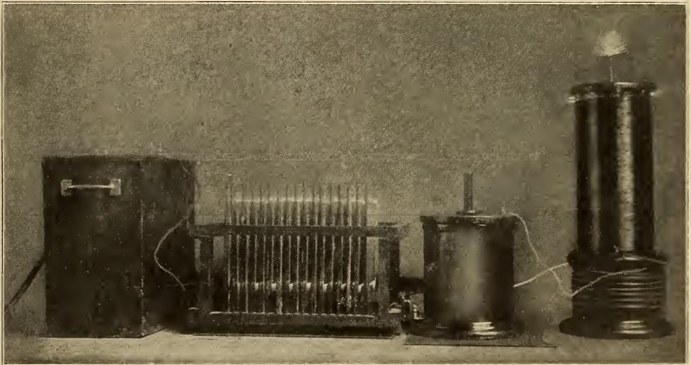
FIG. 1. APPARATUS FOR GENERATING HIGH FREQUENCY CURRENTS.
