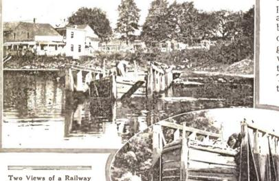
Two Views of a Railway for Carrying Canal Boats Up a Mountainside. The Canal Boats Float Into a Cradle Mounted on Wheels and Are Then Hauled Up the Incline by Means of a Cable.
