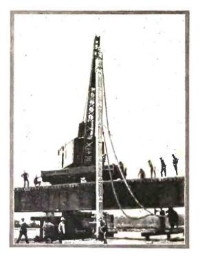
The Many Difficulties of Pile-Driving Have Been Eliminated in This New Pile Which Bores Its Own Hole.
