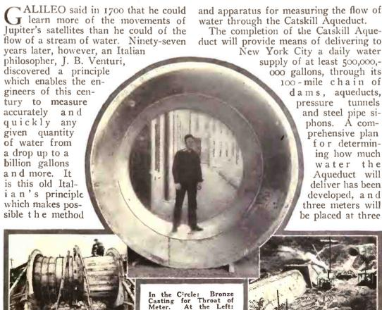
One of the Meter Throats. At the Right: Section in Aqueduct Line Reserved for Meter. points in the line, so that a continuous record of the actual flow will be available.
