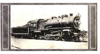
The Third Atlantic Type Locomotive Used Was in Reality a Freight Engine Boiler Mounted on Passenger Engine Wheels.
