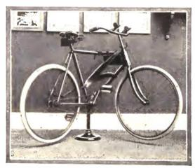
One of the Folding Bicycles used in the Swed.sh Army, which can be Folded and Carried on the Soldier's Back by Means of a Strap.
