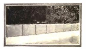
An Enterprising Property Owner has Made Good Use of Discarded Sidewalk Slabs by Using Them as a Retaining Wall.
