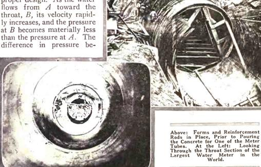
tween A and B can be accurately measured, and bears an exact ratio at all times to the flow through the throat B.
