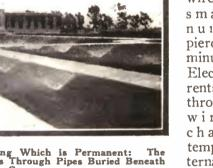
A System of Lawn Spraying Which is Permanent: The Water is Fed to the Nozzles Through Pipes Buried Beneath the Grass.
