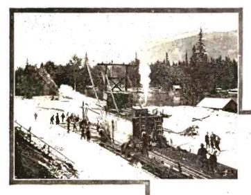
Above: A Track-Laying Machine Working Near the Summit of Yellowhead. In 1913 and 1914 This Machine Averaged Nearly Two Miles of Track Per Day. At the Right: Banks Along the Skeena River, British Columbia, Through Which the Line Was Built.
