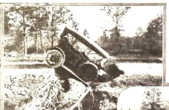
Two Views of a Strange Accident that Befell a Powerful Touring Car. Although the Automobile Made a Large Hole in the Ground, the Only Damage it Sustained was in the Form of a Bent Front Axle and Damaged Front Mud Guards.
