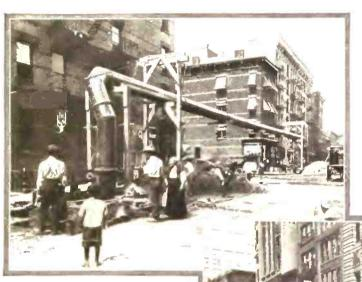
Two Views of the Wooden Trestles Which Carry the Gas Pipes Over the Streets During the Construction of New York's Subways. These Overhead Pipes Have Eliminated the Danger of Explosions Due to Leaking Pipes.
