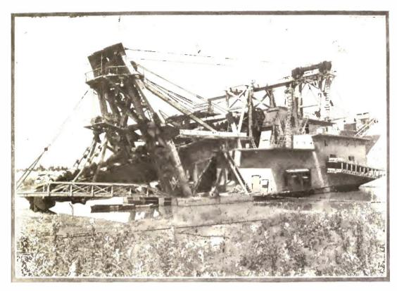
Claimed to be the Largest and Most Powerful in the World, this Dredge is Being Used in California for the Recovery of Gold. The Dredge has 87 Buckets of 16 Cubic Feet Capacity Each and is Electrically Operated.
