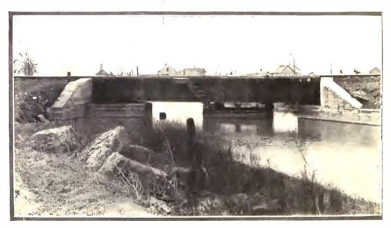
A Drawbridge Which is So Constructed That Trains May Pass Over it at Full Speed. It Requires One Man About Half an Hour to Open and Close the Bridge.
