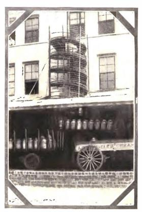
Much Time in the Handling of Milk Cans is Effected with the Use of a Spiral Can Slide.
