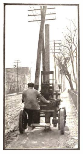
The Gasoline-Operated Tamping Machine is a Recent Addition to the Ranks of Labor-Saving Devices. It Does the Work of Several Men.
