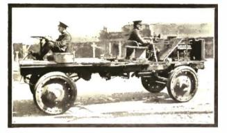
To Allow Greater Flexibility of Action, Recent Canadian Armored Automobiles are being Fitted with a Double Set of Controls.
