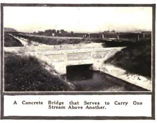
gles to this ditch are a number of natural storm drains. It was desired that the water from these storm drains should not empty into the main ditch and to avoid this these bridges were construct-
