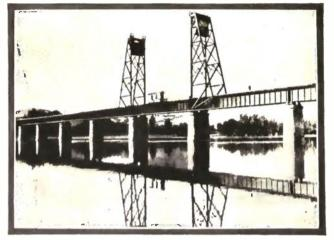
The Lifting Power of this Deck Girder Bridge is Furnished by a Gasoline Engine.
