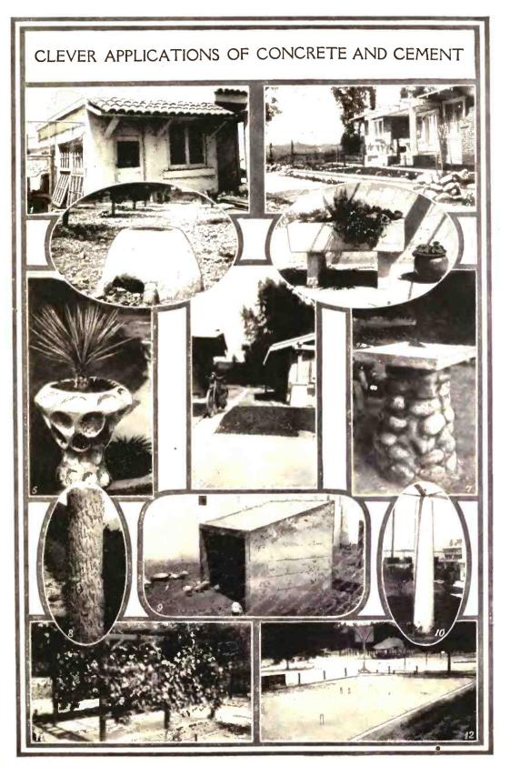
of a cement enclosure wall is a practical application and can be very easily built. The wall is about twelve inches high and four inches thick.
