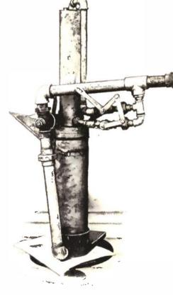
By Means of This Device it is Possible to Inject Ballast Under Railroad Ties After the Track has been Lifted.
