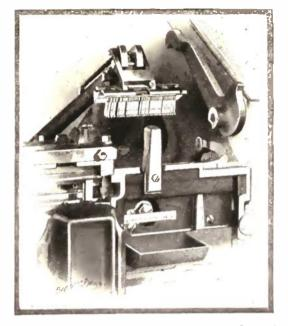
The Elevator Arm in the Act of Taking a Line of Matrices which are to be Carried to the Distributing Mechanism.
