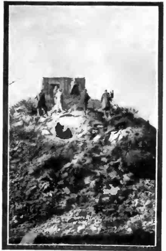
Laborers Digging Great Holes in the Side of the Hill in Which the Explosive Was to Be Placed.
