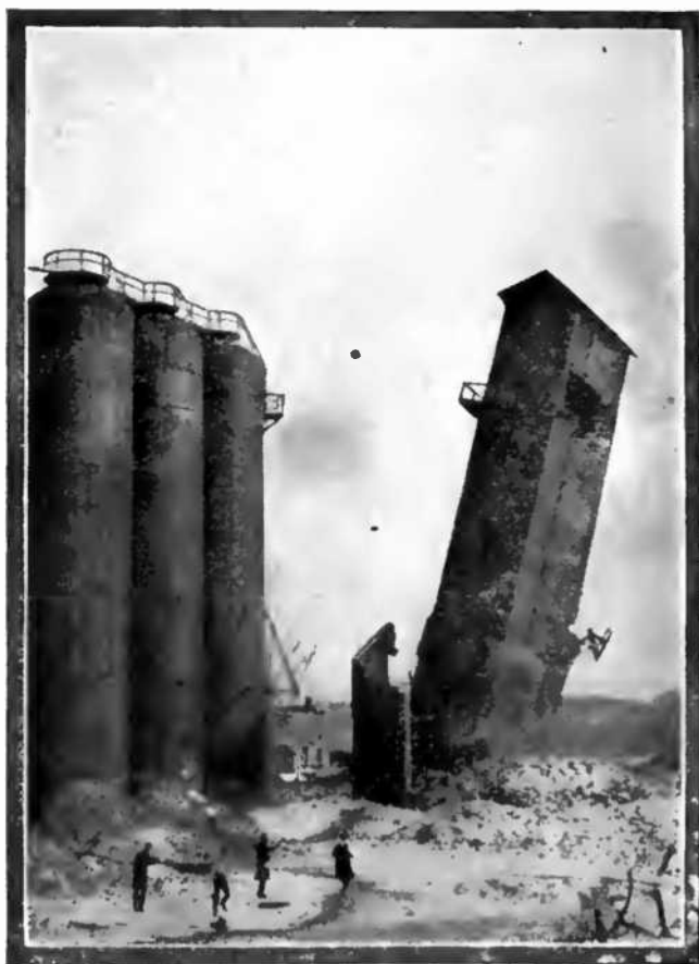
Wrecking an Elevator by Means of a Cleverly Placed Dynamite Charge.
