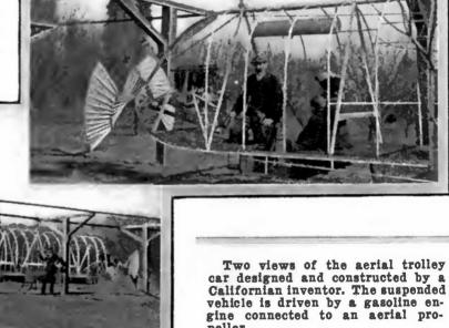
having two fan-shaped blades of sheet metal on ribs of steel tubing.
