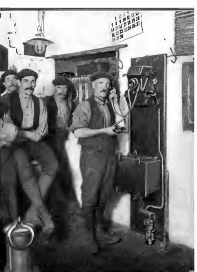
In Many German Mines a System of Wireless Telephony is Employed; the Rails and Pipes through the Mine Conveying the Current Between the Instruments.
