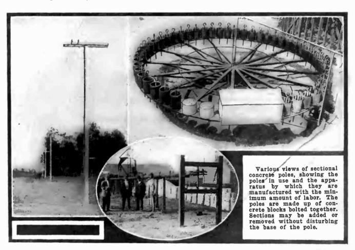
collecting the blocks after they are cured. The wheel is also provided with automatic sprinkling devices by which the blocks may be moistened with water while they are curing.
