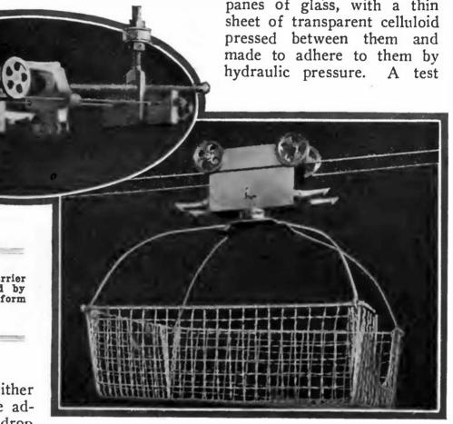
Two Views of a Cash Carrier System which is Operated by Small Electric Motors that form Part of Each Carrier,
