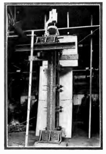
By Means of this Machine, Continuous Brass Tubing can be Made with No Other Attention than to Furnish the Metal.
