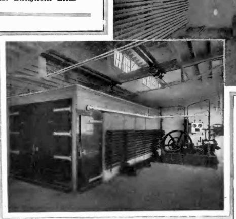
Above: The Interior of a Refrigerator Room in which an American Automobile Manufacturer Tests his Cars.
