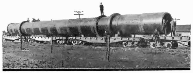
Four Cars Were Required to Haul this Steel Tube Measuring 120 Feet in Length and Weighing 149,000 Pounds.
