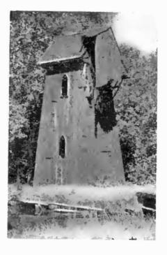
After the Water has Passed Through the Turbine Wheel of the Mill, it Drives the Wheels of this Tower. A Cable Transmits the Power to the Mill.
