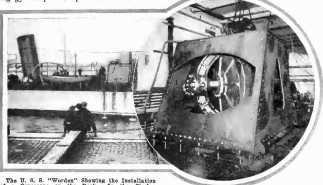
The U. S. S. "Worden" Showing the Installation of a Gyroscope on the Deck. In the Circle: Method of Mounting a Gyroscope on Shipboard.
