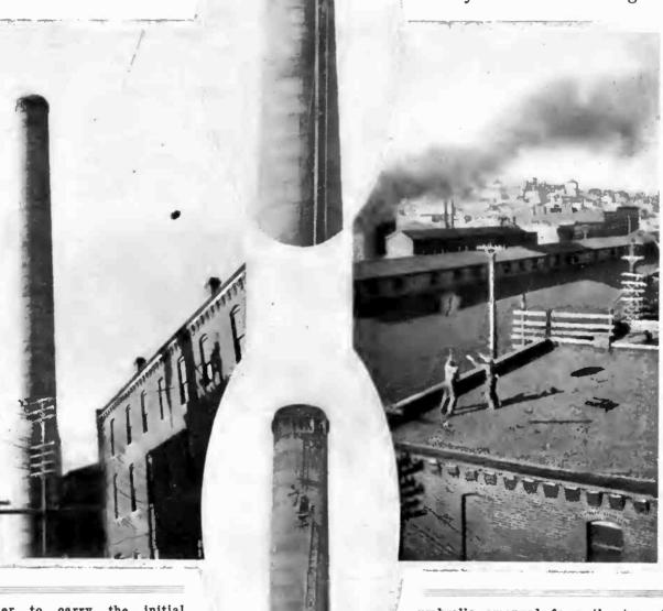
In order to carry the initial string to the top of a tall chimney, a rather novel method was employed. The string was fastened to an umbrella that was placed in the stack so as to be pushed upwards by the heated gases. The
