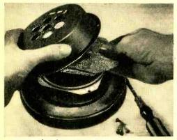
pattern of holes. Coat the inside and outside of the plate with an air-dry wrinkle varnish. Back the perforations with several thicknesses of bronze window screening. The mounting board may be simply a piece of wood to which the pie plate is screwed, or, preferably, it can be a disc of wood turned on a lathe to accept the lip of the pie plate. -D, D, V.
