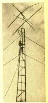
"Spike," K2OKG, constructed this 32' tower (from plans in POPULAR ELECTRONICS, November, 1956) to support his 15-meterrotary "quad" antenna.
