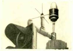
can be avoided. The solution has been provided by Electronic Protection, Inc., with a system of radio-controlled traffic lights. A signal from any emergency vehicle will turn all lights against traffic so that the vehicle can safely pass.
